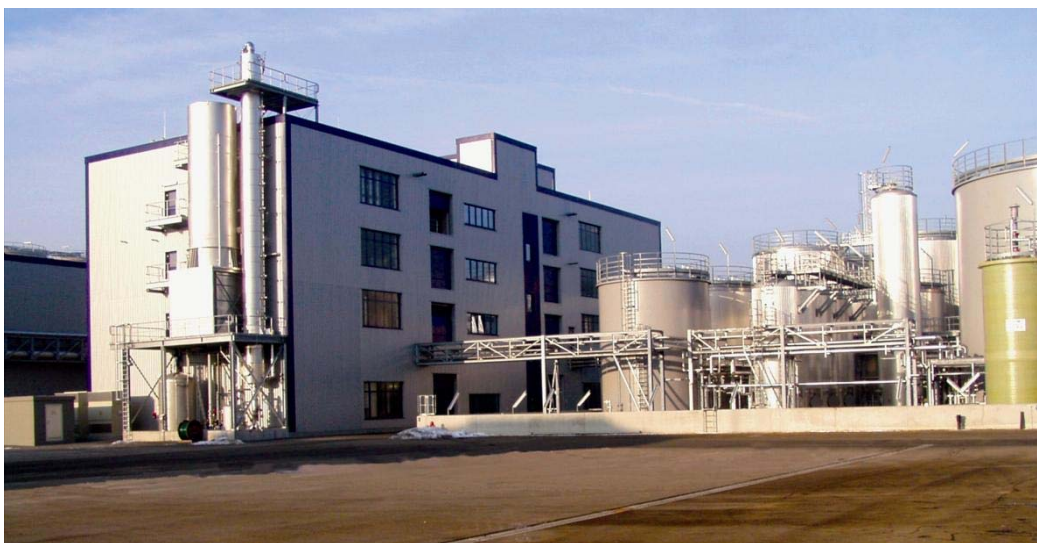
Fig. 1: Verbio Diesel Schwedt – a biodiesel process plant with 100% PROFIBUS
